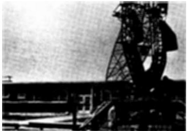
Figure 4. Height finder radar located near ground level.
